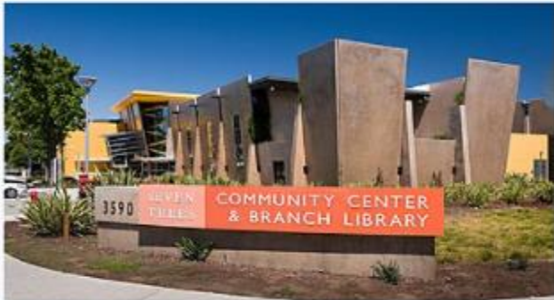
Seven Trees Community Center and Library, part of the San José Public Library
